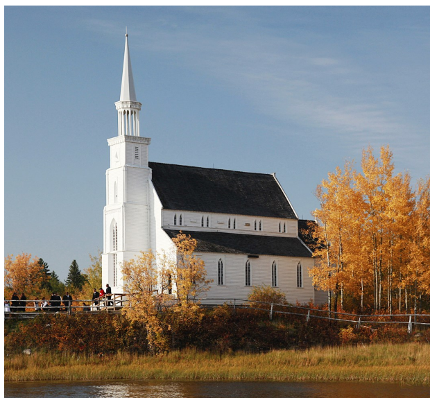
Holy Trinity Anglican Church at Stanley Mission is the oldest standing building in Saskatchewan, built between 1854 and 1860.
